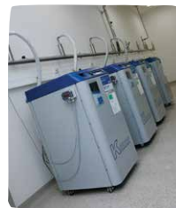
Maintenance & Mechanic Rooms
